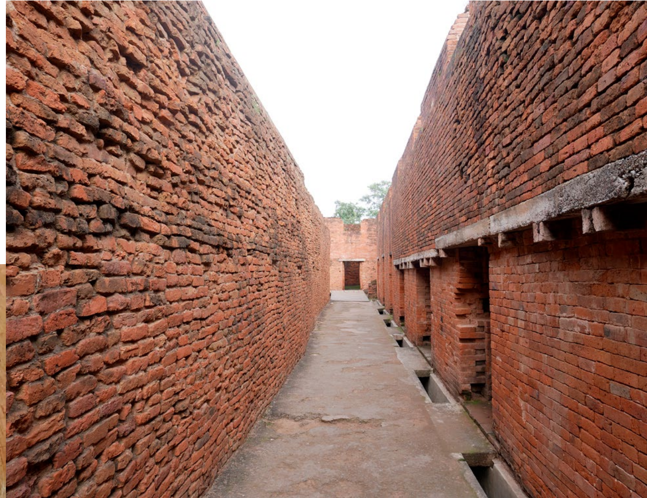
View of the corridors of the University with rooms and sewage ducts
